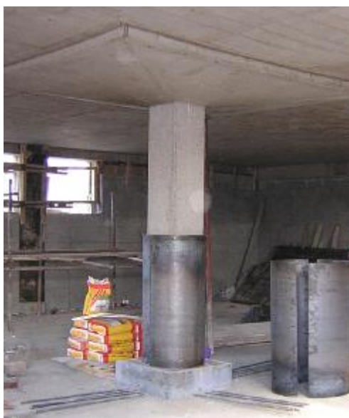
Slika 5. Ojačavanje stuba čeličnom cevi Figure 5. Column strengthening with steel tube
