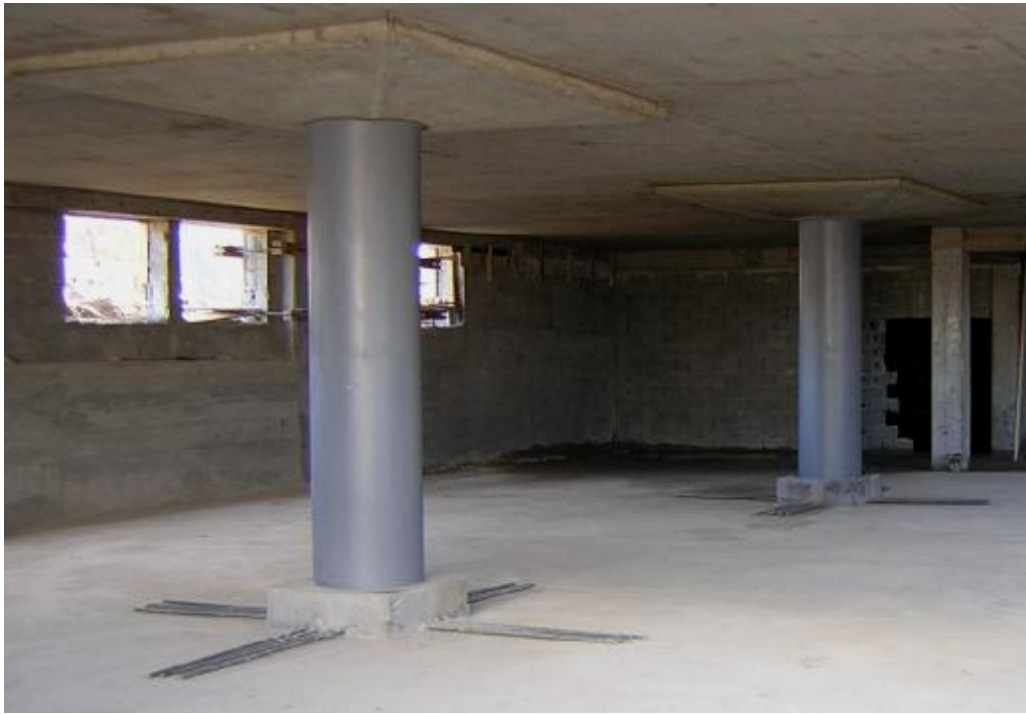
Slika 6. Izgled stubova nakon ojačavanja Figure 6. Final shape of the columns after strengthening
